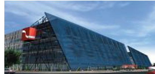
1MW on-grid BIPV System for Suntech's new R&D Center in Wuxi, China
